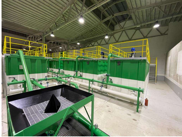
Figure 2: Tanks and piping manage the transfer of products to storage and mixing tanks in the enclosed facility which can operate 24/7 including in bad weather. Solar panels reduce energy costs and contribute electricity to the national grid.
